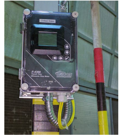
F-4300 Clamp-On Ultrasonic Flow Meter
