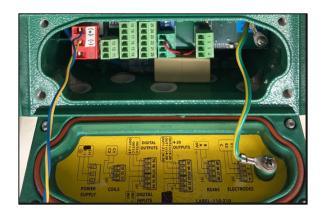
6. Disconnect any existing network cable connected to the transmitter MODBUS TCP/IP adapter (see arrow) and use the patch cable to perform a direct network connection to the transmitter. Note: If your computer only has one network interface, you will lose access to the network, so prepare accordingly and make sure you have downloaded and installed the eSearch utility before proceeding. Also, document the current connection before disconnecting.
